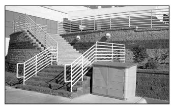
VERSA-LOK units are adaptable to various stair-rail anchoring options.
