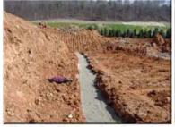
Begin by digging a two foot wide The footing depth will vary based on the the As preparation of the footing trench. Excavate all loose soils and native rock until hard entire weight of the wall.
