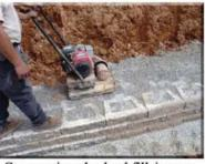
Compacting the backfill is very important. This provides additional resistance to pressures exerted on the wall and prevents settlement. Repeat this process after each backfill.
