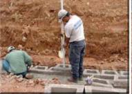
It is always a good idea to shoot grades from time to time to ensure your wall is maintaining the correct level.
