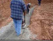
and use a vibrating plate tamp to achieve proper compaction. Get footing as smooth, level, and compacted as possible.
