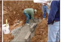
Run a string line for straight walls. This will help in the alignment of the first course. Use a cement trowel to smooth out base prior to setting first block.
