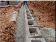
Align and batter each course prior to Angn and batter each course prior to core filling with rock. Batter means setting each course back 1/4 - 1/2 inch behind the course below as seen in the picture above. On straight walls, use a stringline. In curves, visually align the wall to achieve the desired appearance.
