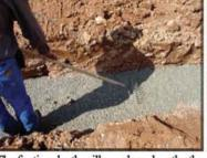
height of the wall. Rule of thumb is 1 inch continues, remove all large rocks of embedded block per vertical foot of wall original ground is reached. The height is required. Place four to six inches footing will be supporting the of crushed rock (#78 or #8910) in the footing and level for the wall foundation.
