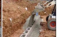
It is recommended that the cores of the block be filled with a #67 or #78 stone no less frequently than every three courses. This same stone is recommended for the backfill as well.
